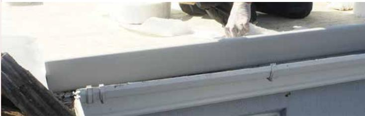
Make sure the laminating roller is used in a controlled fashion (slower) so as not to generate spray.
